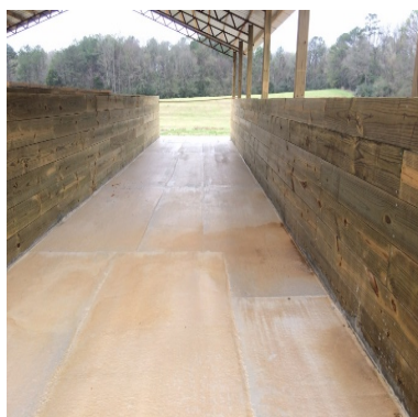
Figure 2. Alleyway composting system.
