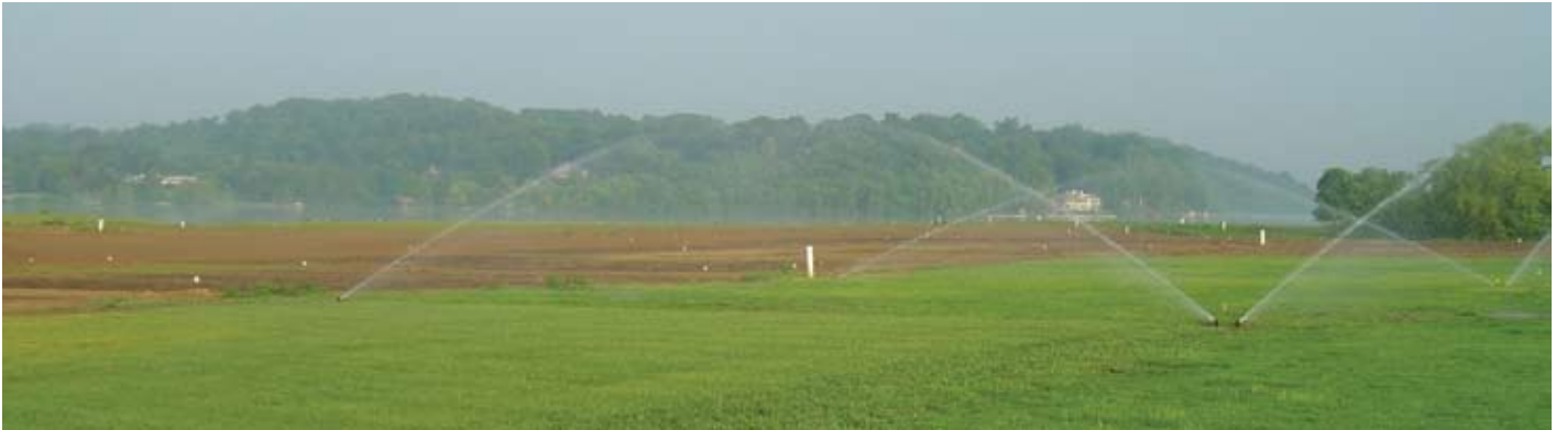
Figure 2. An underground sprinkler system with automatic controller.
