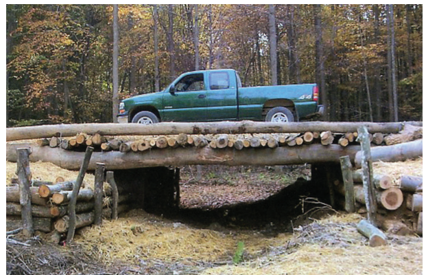
Bridge constructed with on-the-farm materials.
