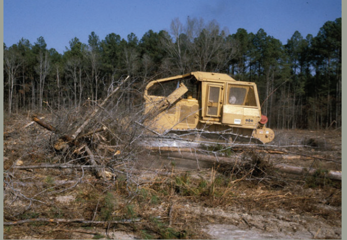
Site Preparation Mechanical
