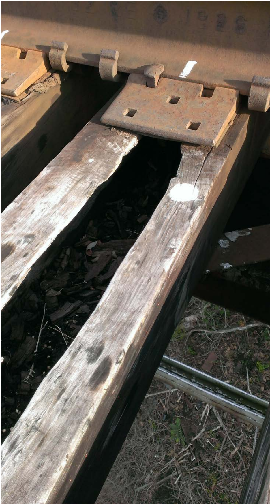
FIGURE 5. Heartwood needs protection, too! The heartwood of this bridge tie has completely rotted away because it is not possible to treat it with creosote or copper naphthenate.
