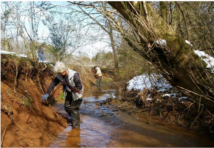
Figure 5. (Left) Volunteers install stakes along an eroded stream channel in a park. (Right) Live stakes hand-driven into saturated clay soils at the toe of the streambank, at a slight angle pointing downstream and at a 90-degree angle to the face of the bank.
