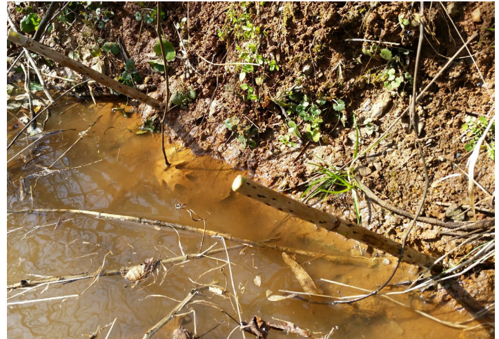
Figure 5. (Left) Volunteers install stakes along an eroded stream channel in a park. (Right) Live stakes hand-driven into saturated clay soils at the toe of the streambank, at a slight angle pointing downstream and at a 90-degree angle to the face of the bank.
