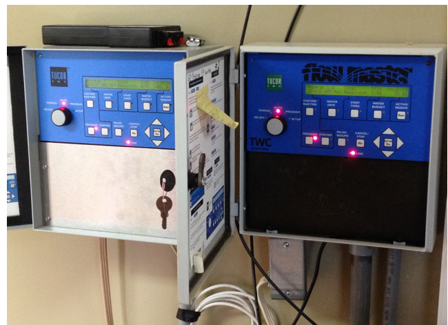
Fig. 4. Irrigation controllers are affordable, low-tech options for reducing manual labor.
