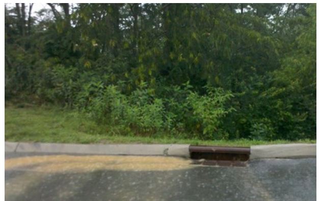
This sediment , or washed away soil, goes through the storm drain and straight into a creek, where it will harm fish and aquatic insect habitat.
