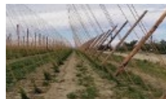
Figure 16: Pole, wire and coir design end row (Washington State hop yard).
