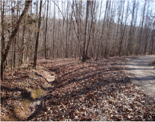
Turnout or wing ditch diverting runoff from the road
