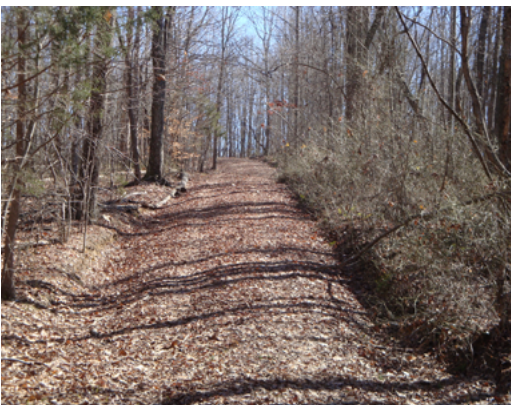
A crowned forest road with ditches for drainage
