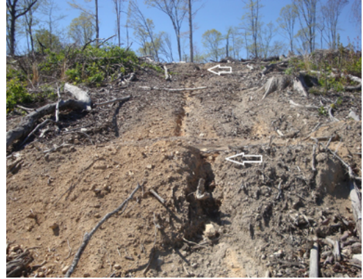
Poorly constructed water bars that are breached causing substantial erosion on a skid trail.
