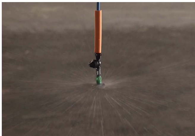
Figure 4. Activated sprinkler in operation.
