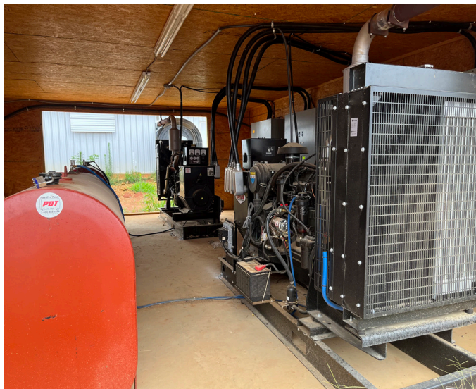
Figure 2. Newer poultry farms often have two stand-by generators and automatic transfer switches, each wired to carry half the load for each house, which greatly reduces the risk of catastrophic flock losses.
