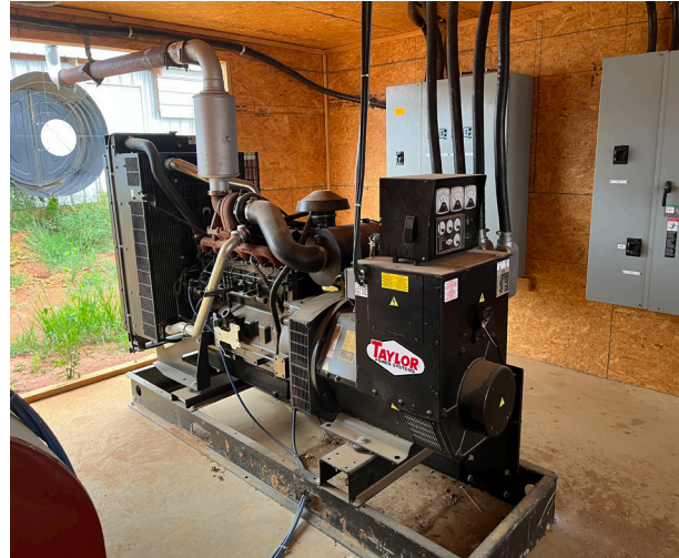
Figure 3. A stand-by generator (foreground) and automatic transfer switches (background) must receive proper maintenance to perform efficiently when needed.
