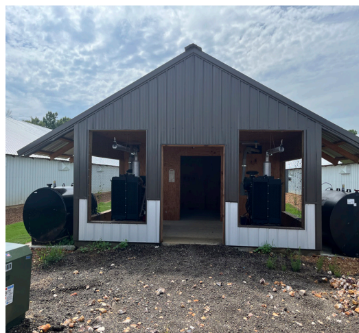
Figure 1. Stand-by generator systems are required for modern commercial poultry farms today. Proper maintenance is critical for the system to provide power at a moment's notice in an emergency.
