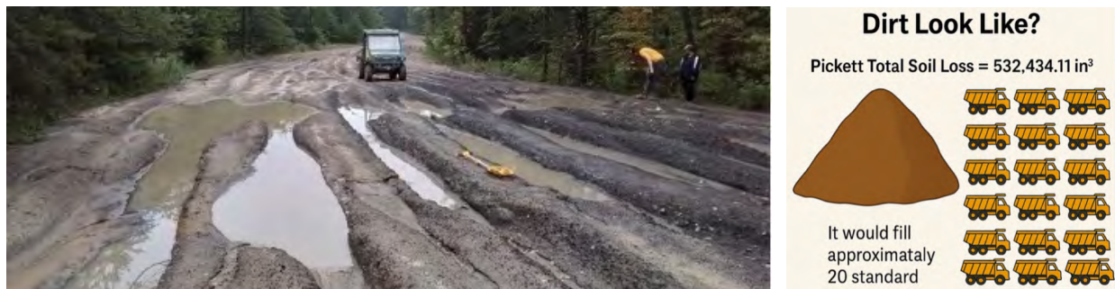
Figure 3: Rutting and water on an OHV trail in Pickett State Forest during ecological assessments.
