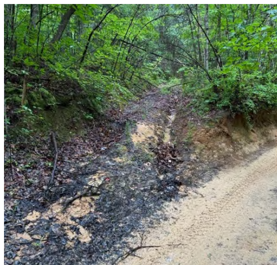
Figure 5: Social trail formed by OHV users driving around a water-filled section of the main trail.
